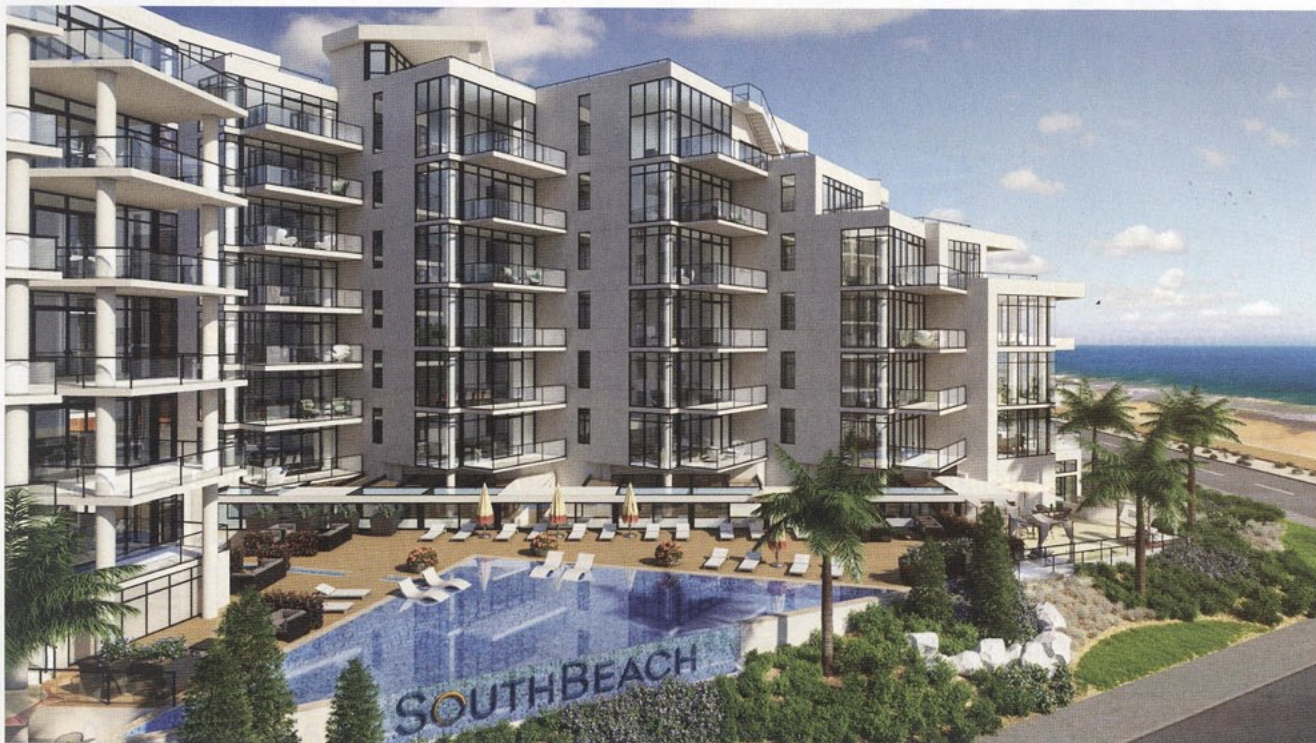
This new five-star, oceanfront, multifamily development in Long Branch, N.J., designed by James Monteforte of Monteforte Architectural Studio, uses Smith-Midland Corp. SlenderWall precast concrete building panels for their aesthetics, light weight, strength, durability, and energy efficiency. Courtesy of Costea Photography Inc.
